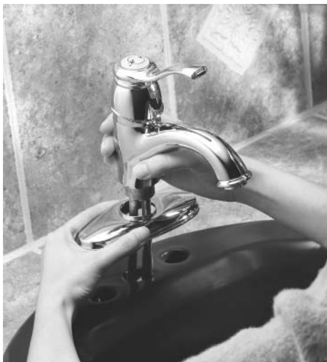
Figure 16.7 Assembling a faucet. Courtesy of Moen, Inc.
